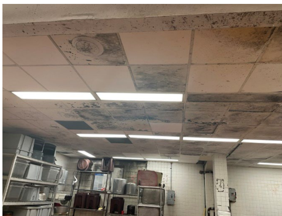
Kitchen Ceiling Tiles
